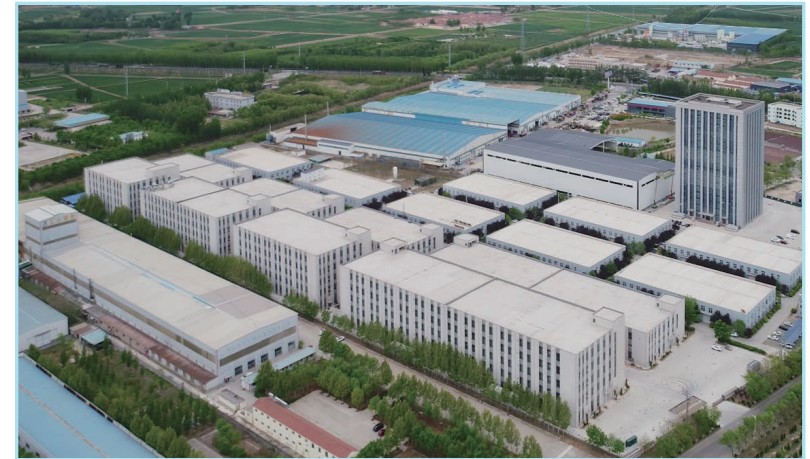
Construction of PSL Phase IV Project in 2021 Factory area 42000 square meters.
